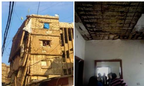
Figure 1-Damaged building, Spalling concrete
