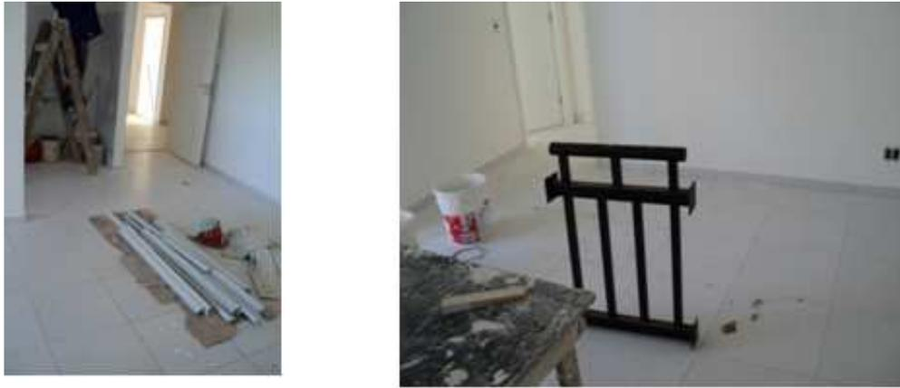
Figure 4: Improper storage of materials
