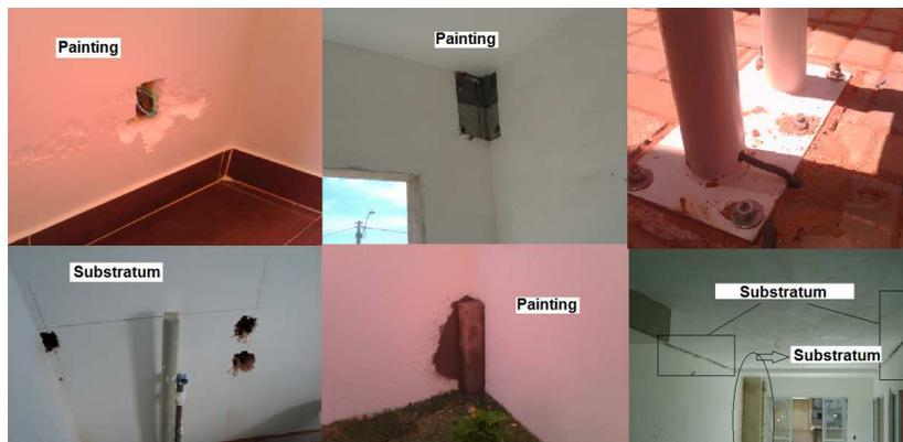
Figure 8: Defects photographic record
