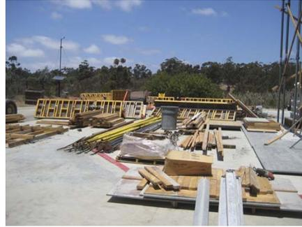
Figure 3: Concrete Formwork Stockpiled in Staging Area near Building
