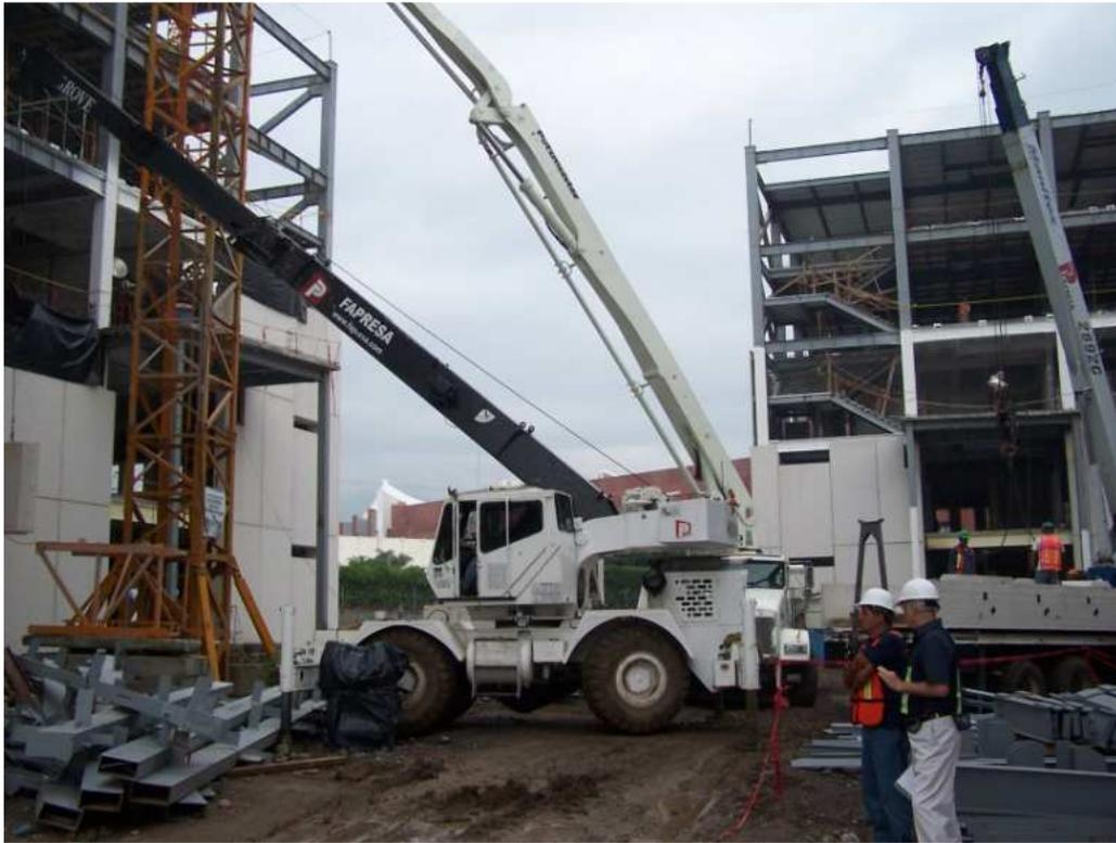
Figure 6: Installation of concrete facades with new sequence
