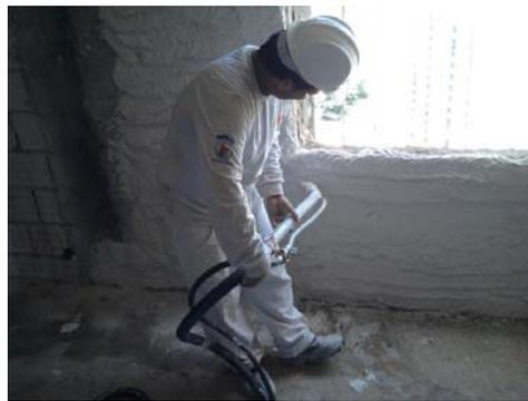
Picture 5 (b): Plasterer projecting gypsum in the wall.
