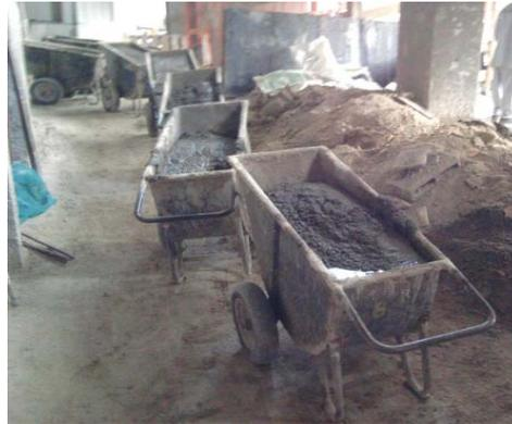
Picture 4 (b): Wheelbarrows in rows in position to get into the hoist.
