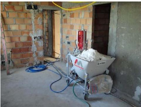
Picture 5 (a): Gypsum machine projector.
