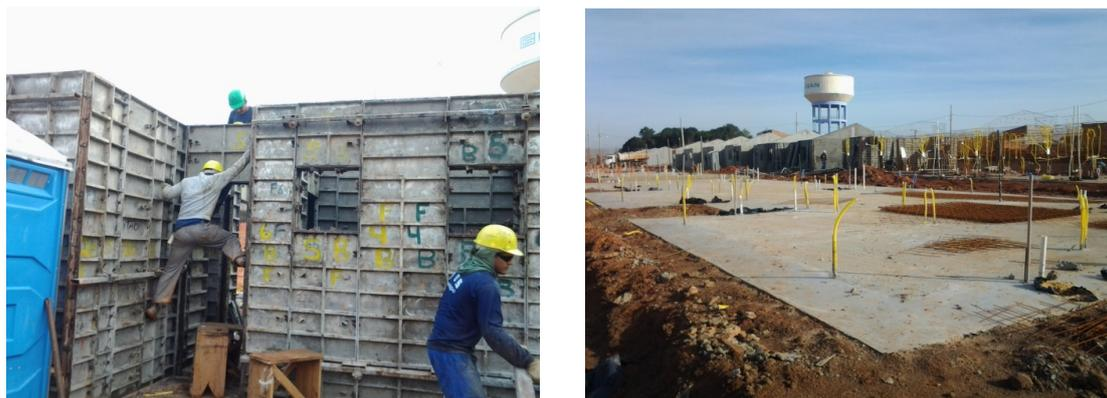
Figure 7: – Examples of improvisation: worker supporting himself on the concrete wall formwork (left) and inadequate electricity pipes in the raft foundations (right)
