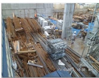
Figure 5: The steel stock at the construction site
