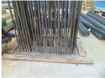
Figure 7: Image of the steel of pillars and the stock of bars on the floor
