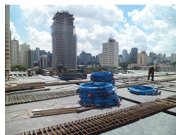
Figure 6: Strands on the floor under construction
