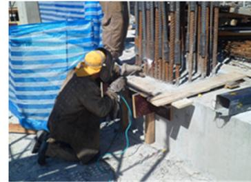
Figure 9: Welding to union the bar of pillars
