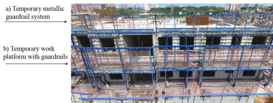
Figure 2: Safety Systems with Guardrails in the Construction Site
