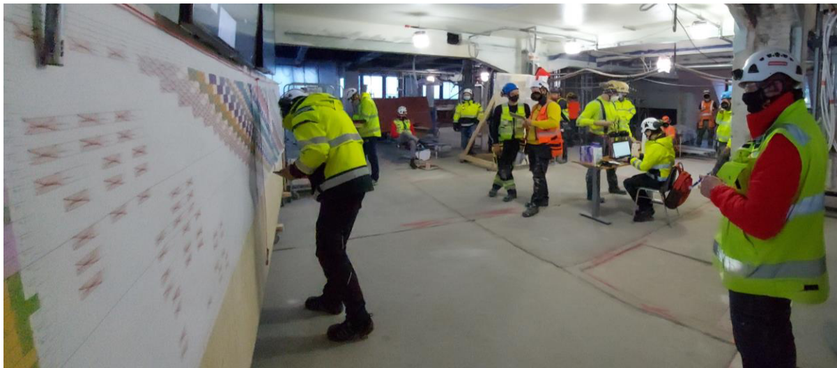
Figure 3: The progress was recorded both digitally and on a visual board in the daily huddles. The raised issues were also recorded in a digital spreadsheet.
