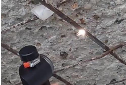
Figure 8: On-site demonstration test situation
