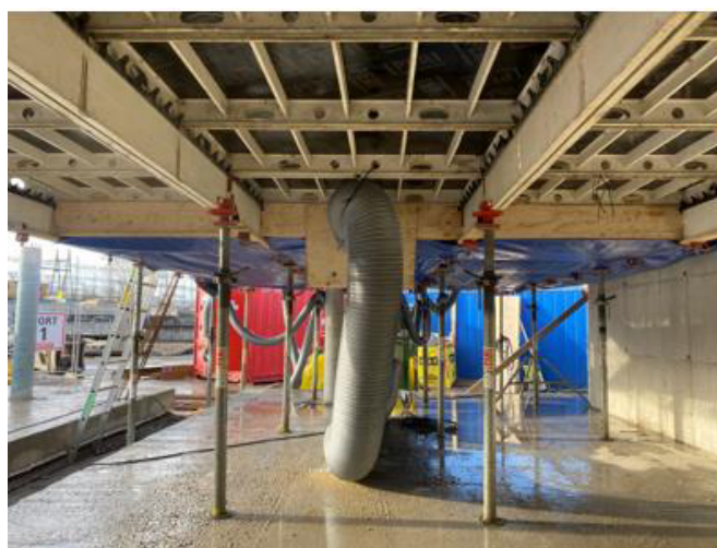
Figure 7: Slab, with hot air underneath
