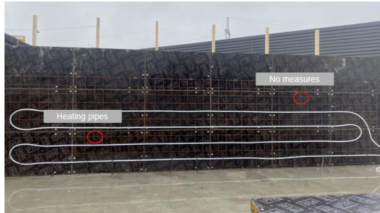
Figure 6: Wall surface, including heating pipes
