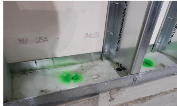
Figure 4: Fasteners Ready and Spray-Painted Green for Inspection
