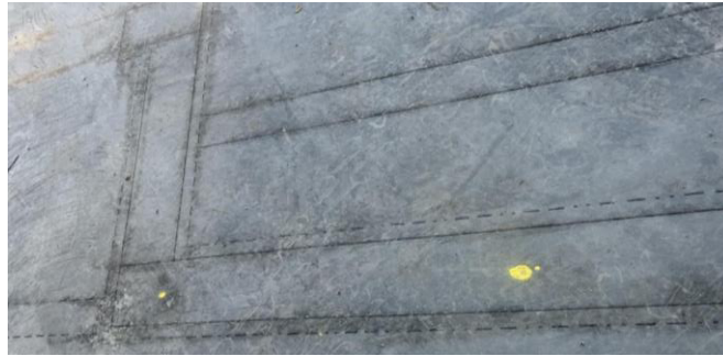
Figure 2: Wall Layout Painted on Floor Slab by Robot
