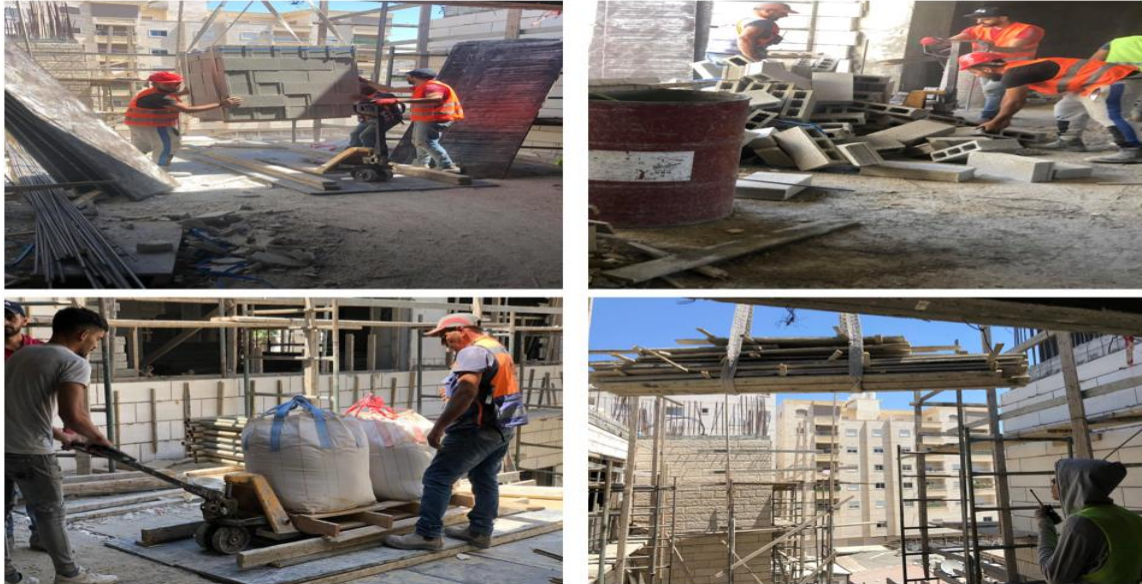
Figure 2: Delivering materials for project C1 using an open balcony
