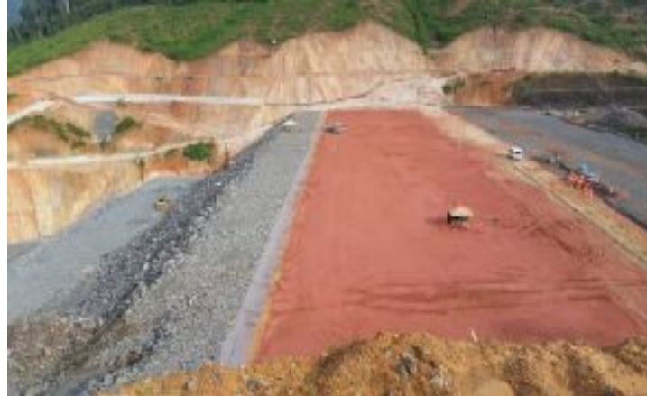
Figure 2: Dam Construction Site
