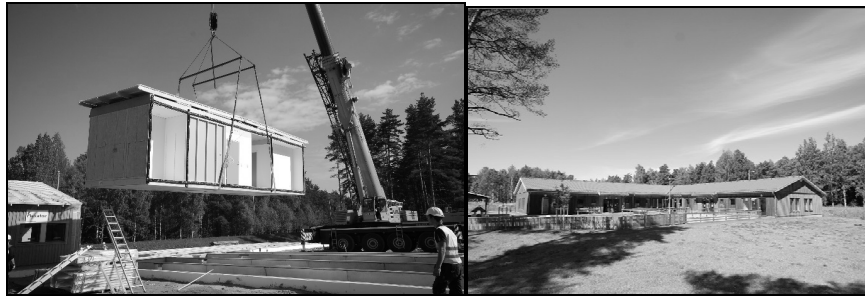
Figure 1: On-site assembly of volume elements and a finished kindergarten project.
