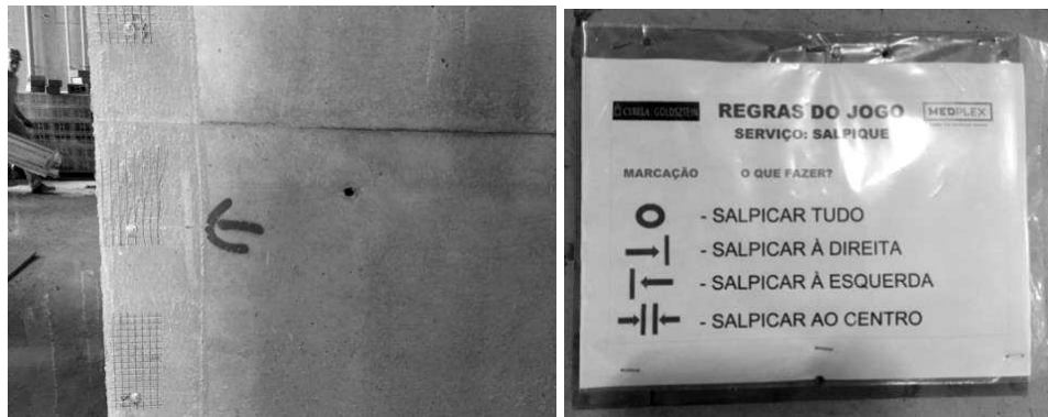
Figure 1: Example of spray marking of the kind of rough cast and its explanatory sheet
