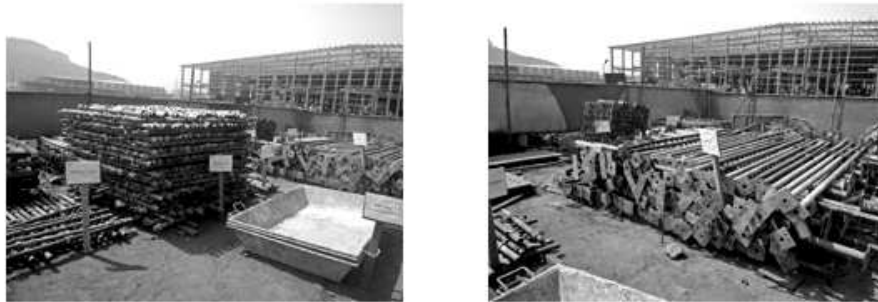
Material storage with labelling
