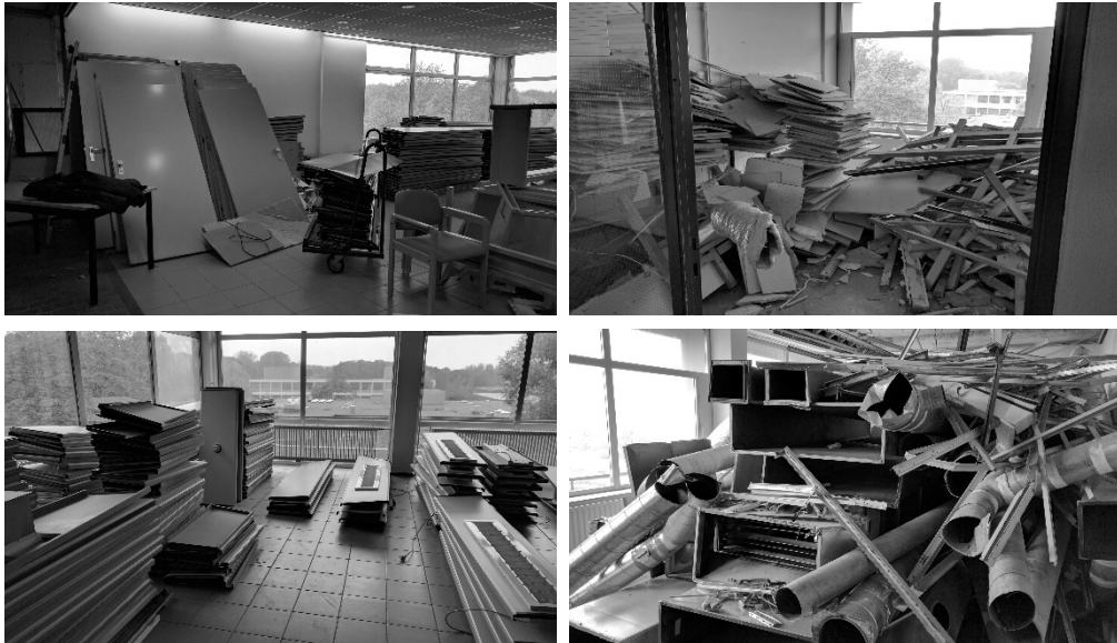
Figure 1: Different Collections of Salvage Elements stored inside the Building updated to a database. On site, elements are dismantled and stored on separate places inside the building (see Figure 1). Nearby customers, whom the company had relations with and who were interested in obtaining the salvaged elements, were invited to the site. In addition, the elements on the database were showcased on the Web-shop.
