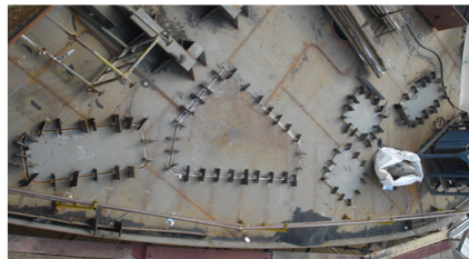
Figure 5 Illustration of outfitting equipment foundations in shipbuilding
