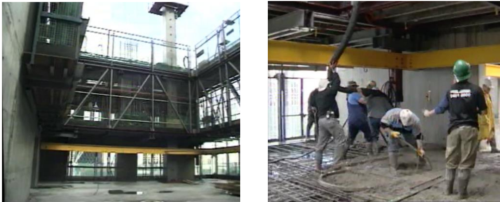
Figure 3: Advanced perimeter system (Double-Jump System, n.d.)
