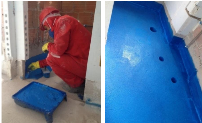
Figure 2 – Waterproofing process with acrylic membrane (courtesy of the company)
