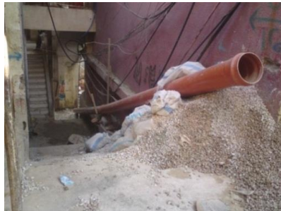
Figure 5: Backfill material delivery
